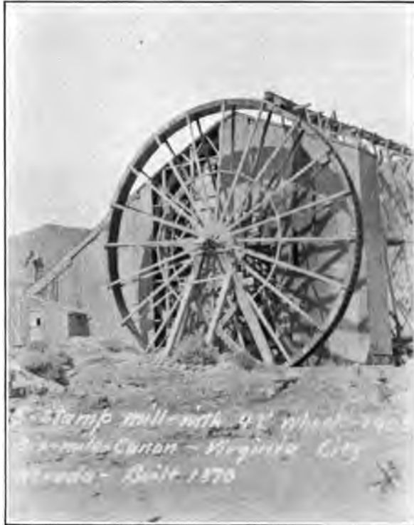
42-foot Wheel, Virginia City, Built 1870
